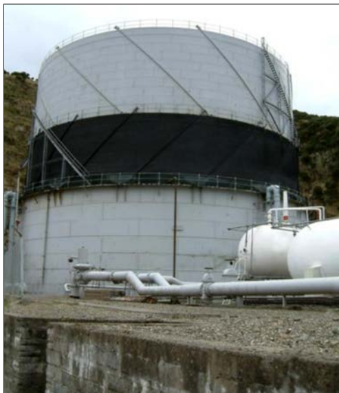
A gasometer, the footprint of which is now a car park
