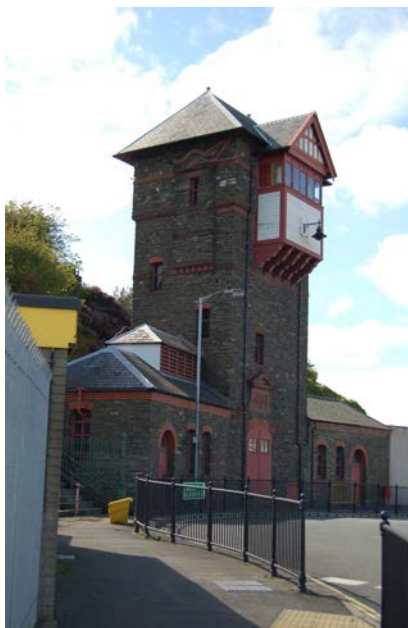
The Bridge Control Building
