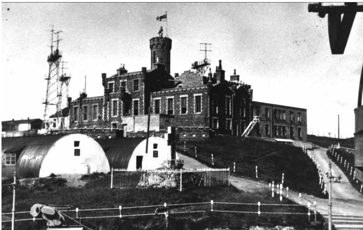
The secret RADAR station on Douglas Head during WWII
