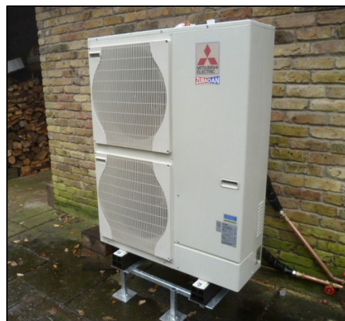
Figure 1: Air Source Heat Pump
