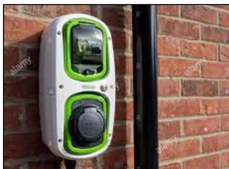
Figure 2: Wall mounted EVCP
